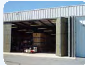
Photos top to bottom: Gunnison Property Core Samples Core shed
