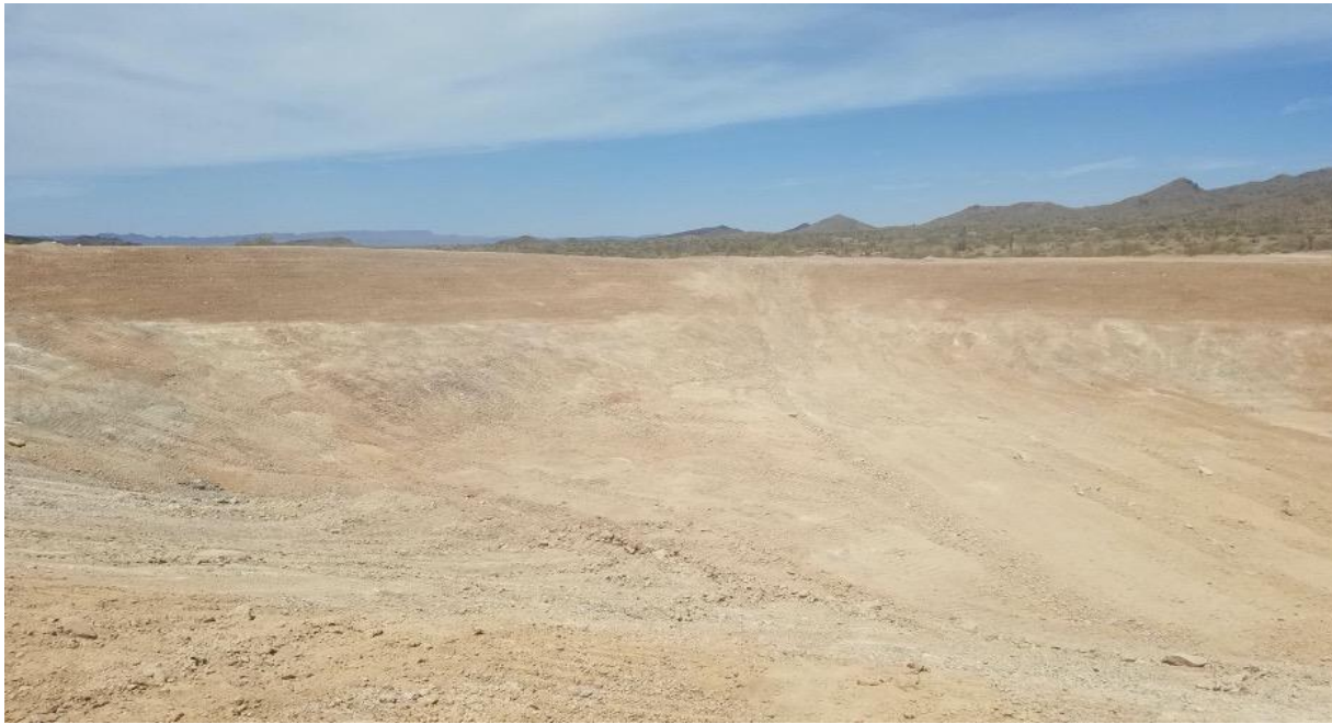
South Side of Leach Pond – Starting Final Grading For Liner
