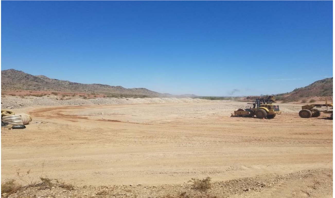
East Side of Leach Pad – Nearing Final Grade
