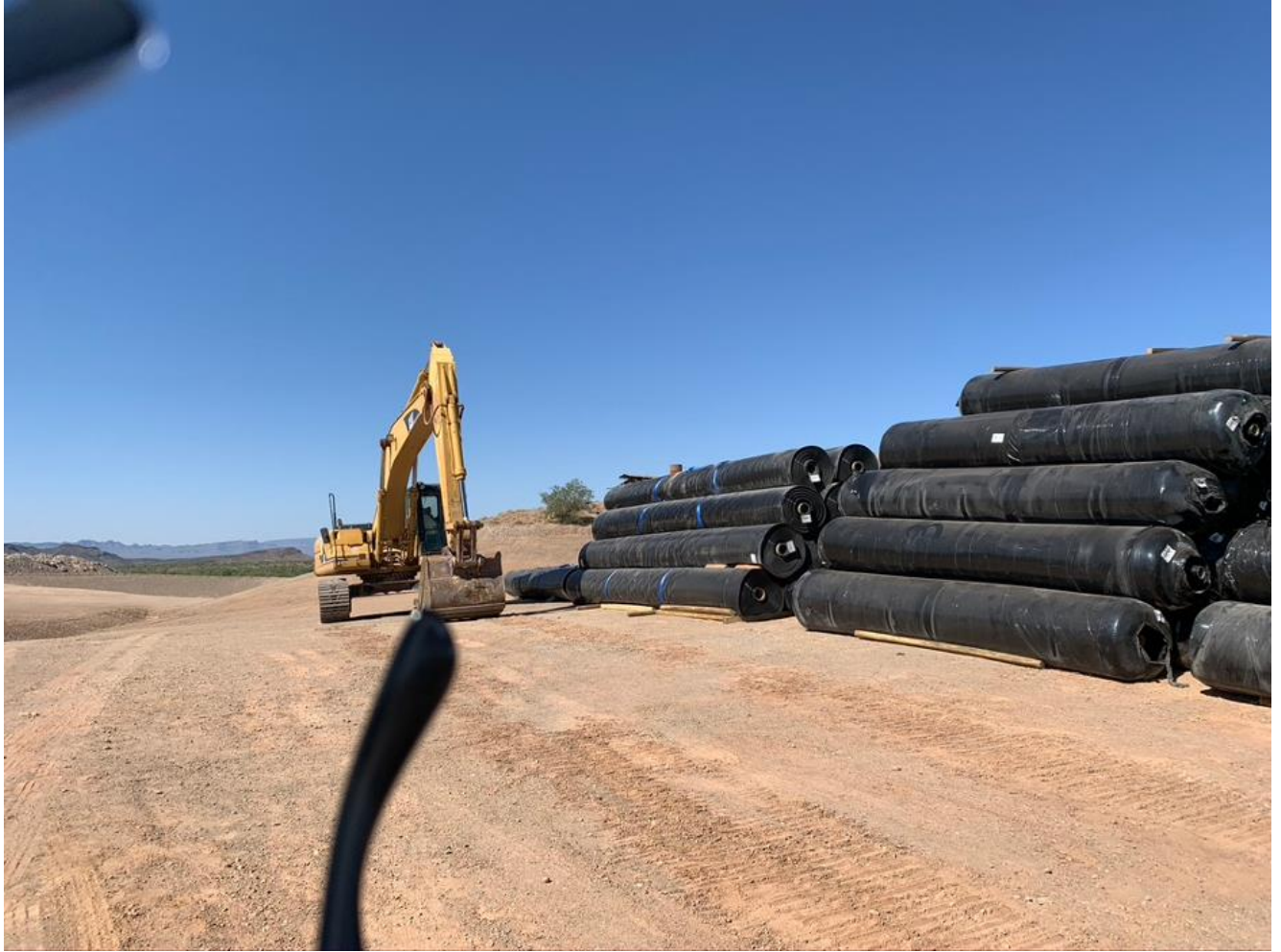
Liner Delivered at Site – Waiting for Install
