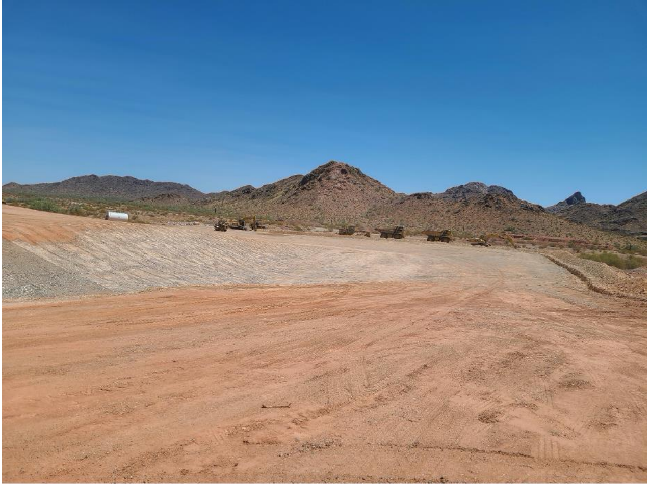
East Side of Leach Pad – Completed Compaction – Ready for Liner
